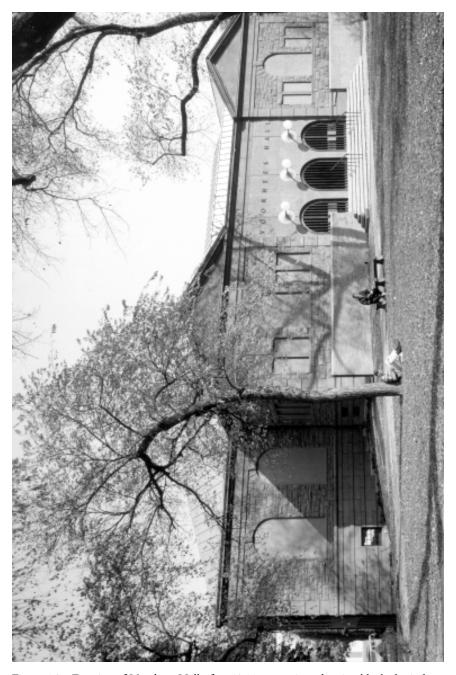
Figure 1.8 Exterior of Voorhees Hall after 1966 renovation, showing blocked windows and new doors. © Victor's Photography, 1967. Rutgers University Photograph Collection, Rutgers University Archives (from Special Collections and University Archives)
